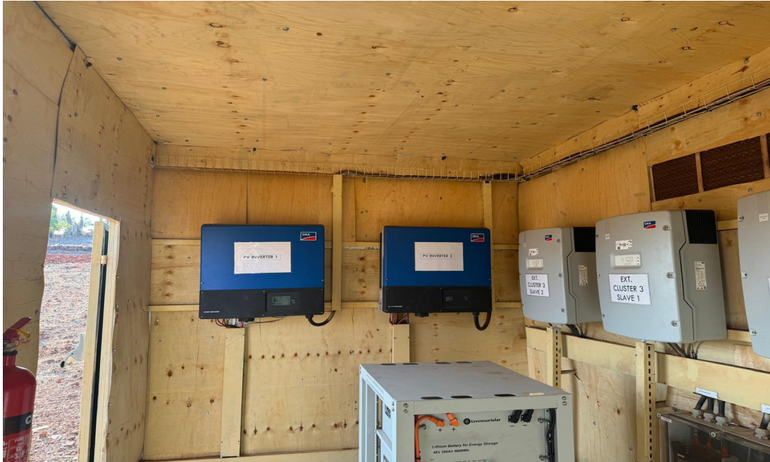
Fig 7: Battery replacements at Arabia
