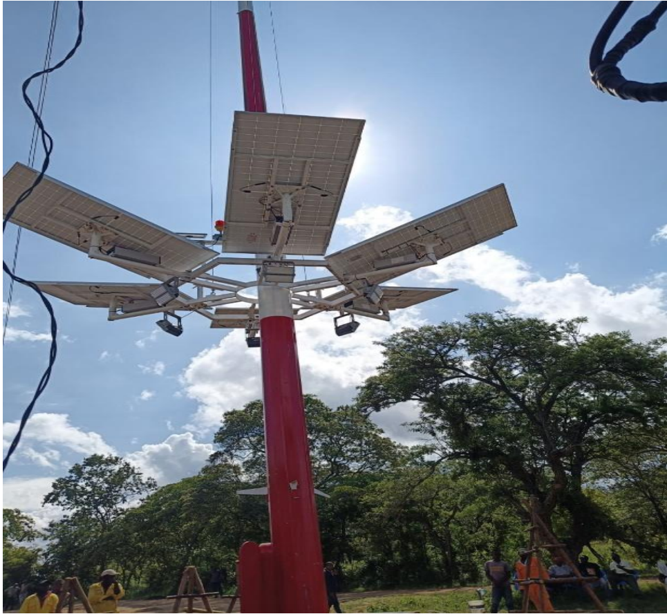
Fig. 5: Testing of solar highmast
