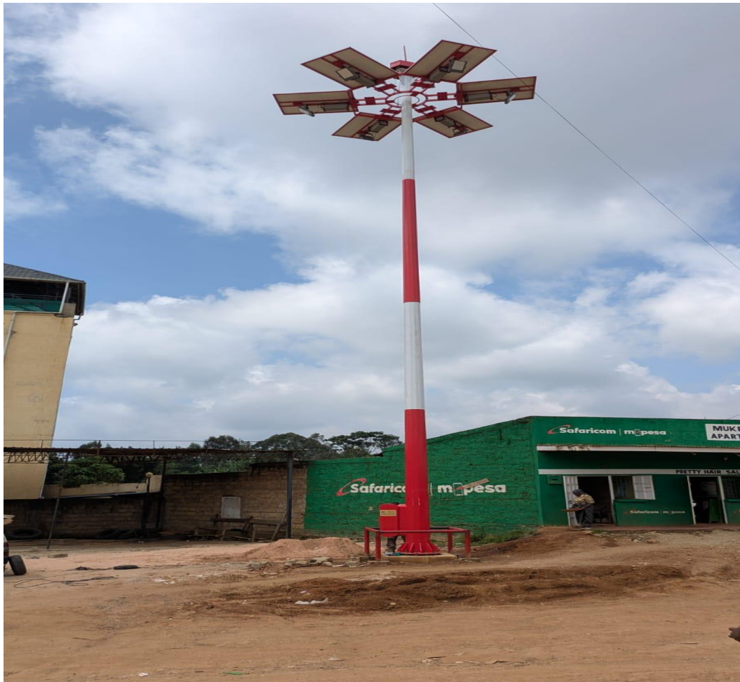
Fig 3: Solar highmast
