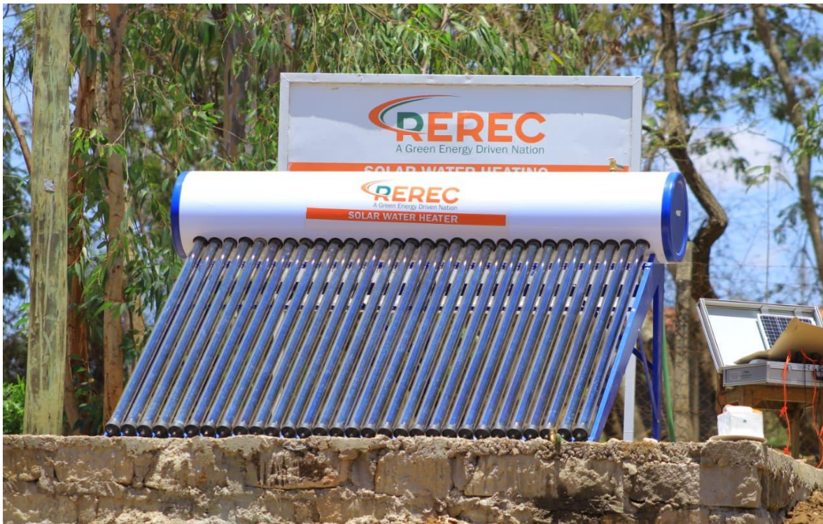
Fig 3: Solar Water Heating System
