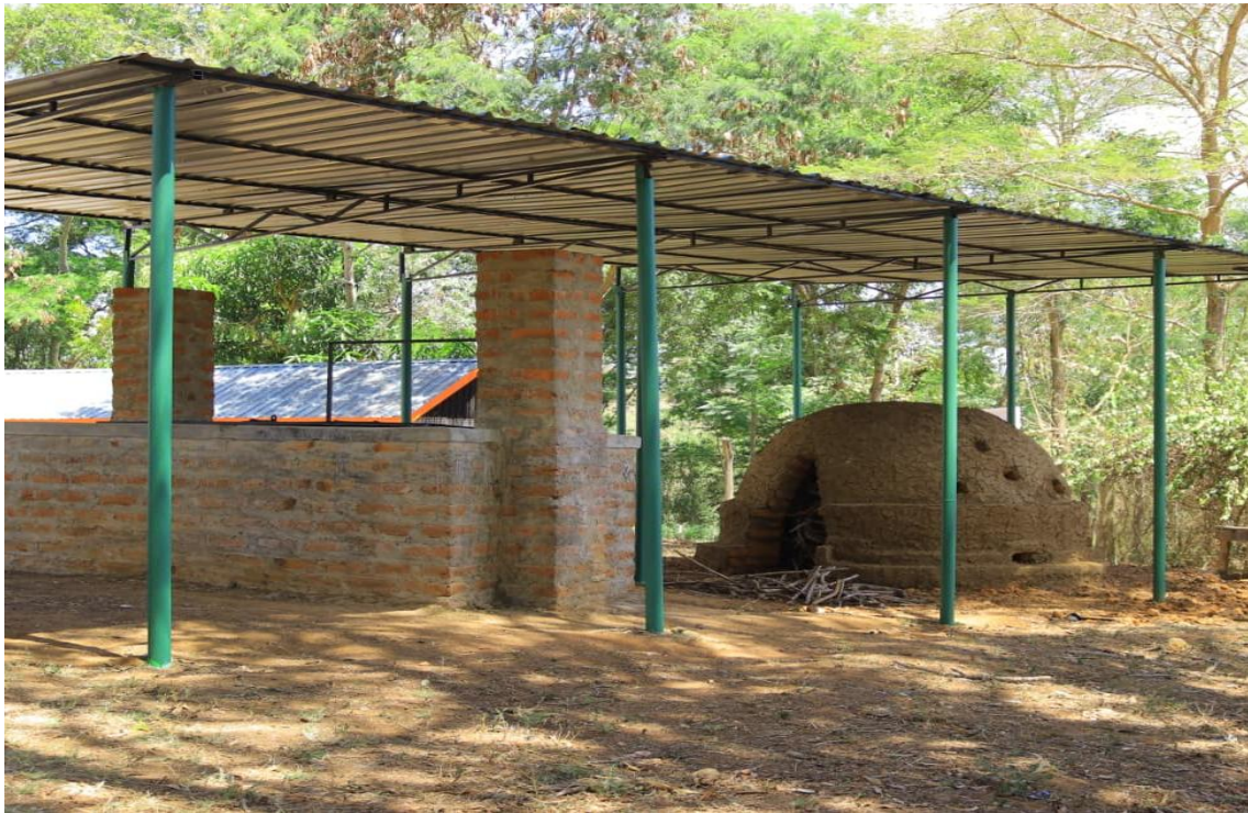
Fig 5: On-Site liners kilns
