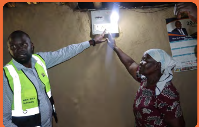
Residents of Essere Village celebrate improved access to electricity through the Last Mile Connectivity Programme.
